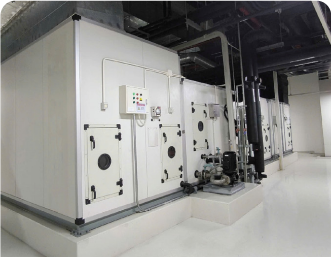
AIR HANDLING UNIT (AHU)
